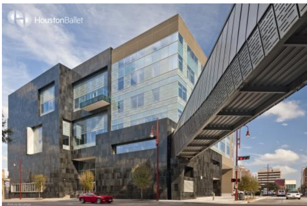
Houston Ballet Center for Dance Building Photo: Nic Lehoux
